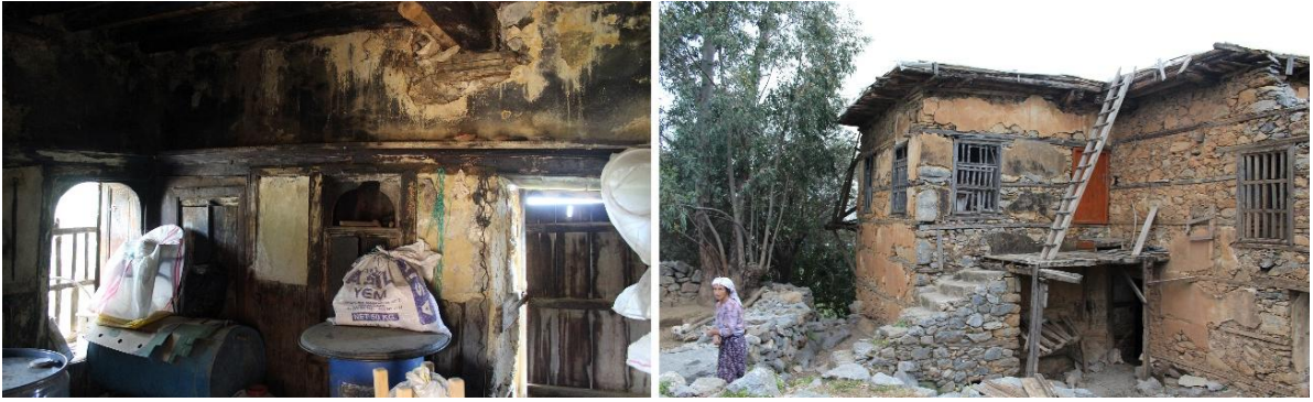
Figure 17. Building Interior Detail and Building Entrance
