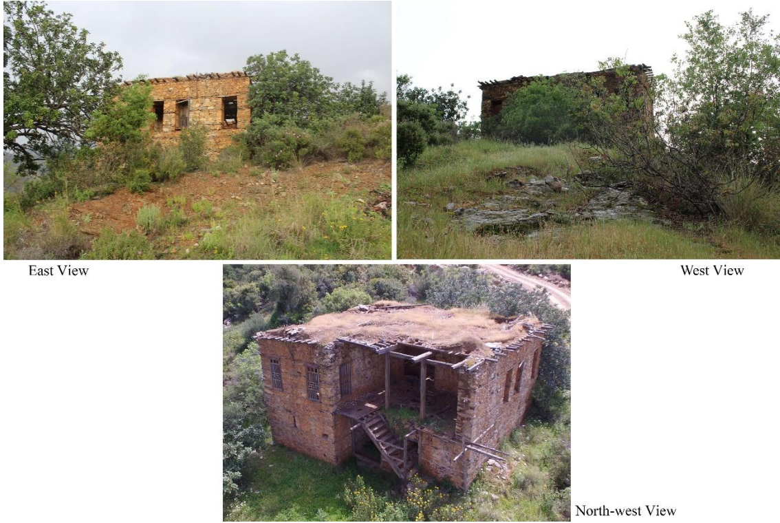
Figure 3. Residence of Halil Agha, the Madrasah Scholar, East, West and Northwest Views
