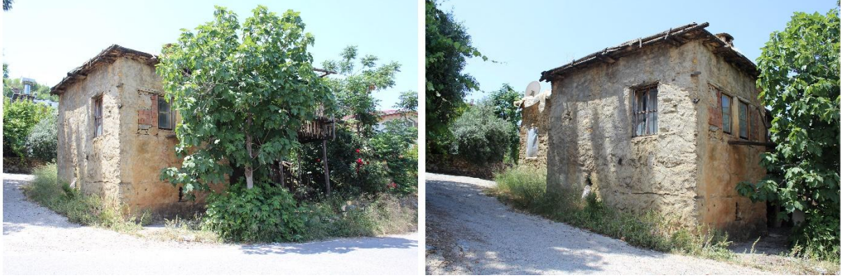
Figure 14. South and West Views
