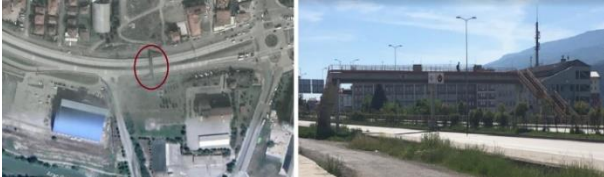
Figure 5. Gendarmery zone overpass satellite photo and terrestrial photograph
