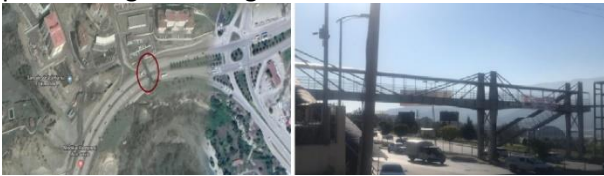
Figure 4. General directorate of security overpass
