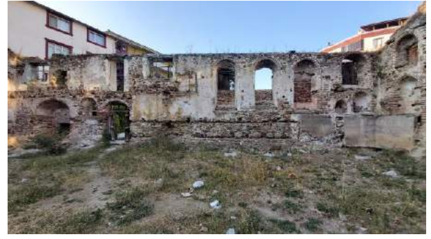
Figure 11. Apertures in the north wall of Azize Paraskevi Church (Personal archive, 2021)
