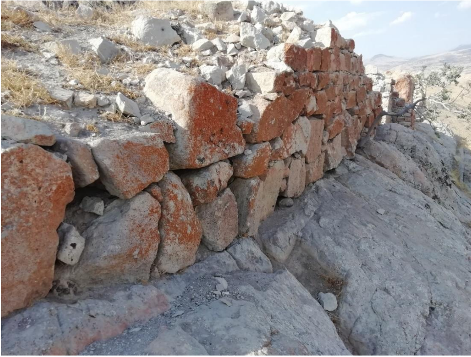
Photo. 3: The East Fortification Walls and the city wall bed on the parent rock.
