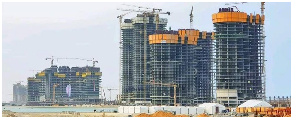
Figure 5. New Alamein City waterfront under construction towers [6]
