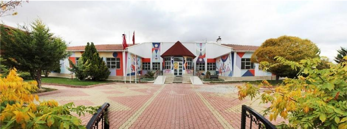
Figure 34. Back Yard Entry View
