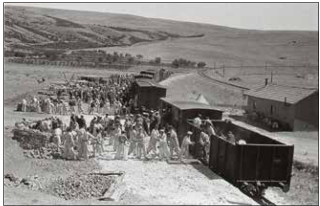
Figure 17: Transferring bricks at Lalahan Railway Station (IHTBV). / Tuğlaların Lalahan Tren İstasyonu'ndan transferi (IHTBV)
