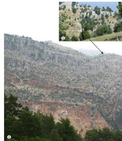
Figure 10. Secondary retrogressive landslide generation within the old slide mass (a) and tension cracks on the upper bound of the landslide (b).
