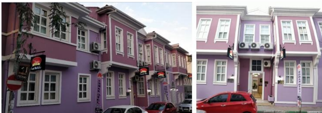
Figure 25. Post-restoration of the buildings
