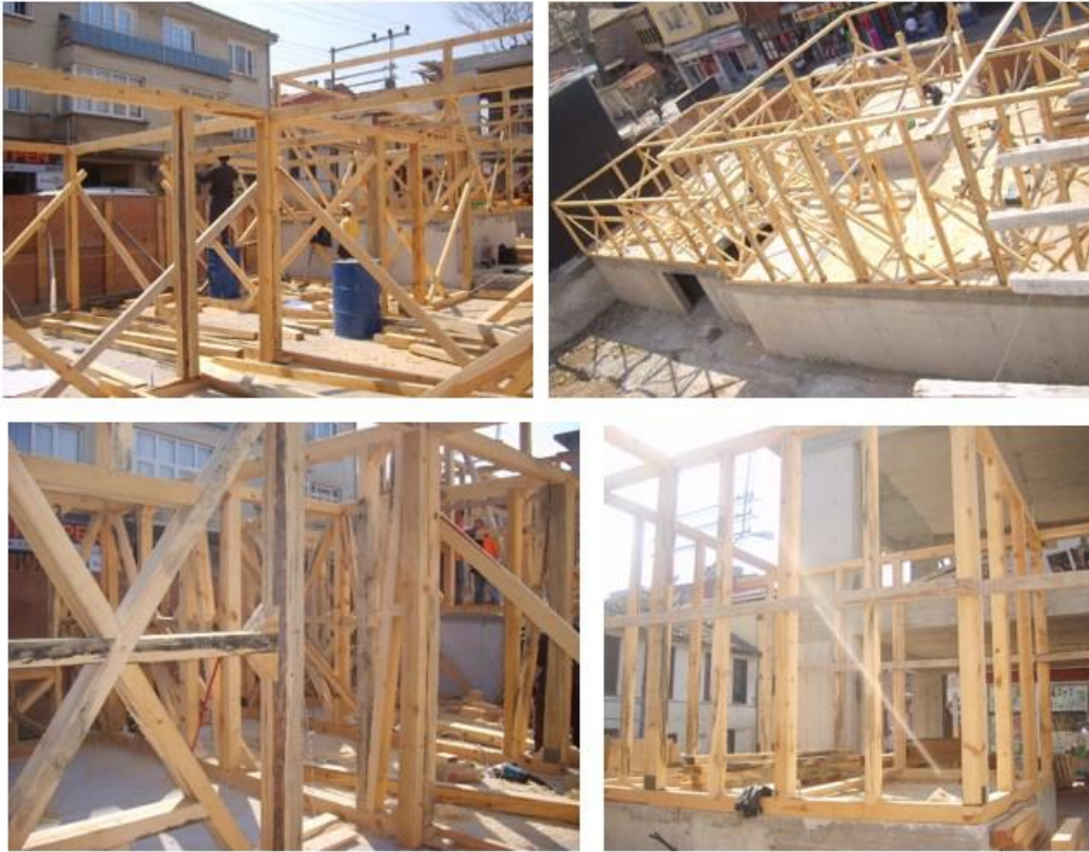
Figure 20. Constructing of the structures in parcel numbers 9 and 10 with traditional techniques
