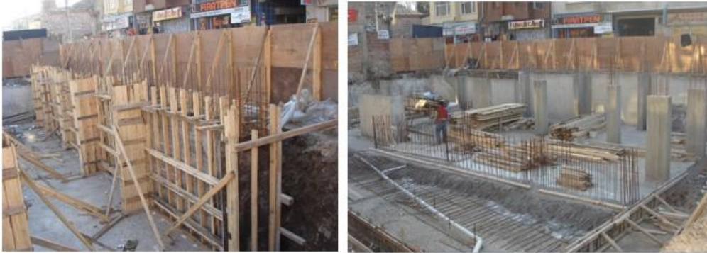
Figure 18. Construction of the foundation of parcels numbers 9 and 10
