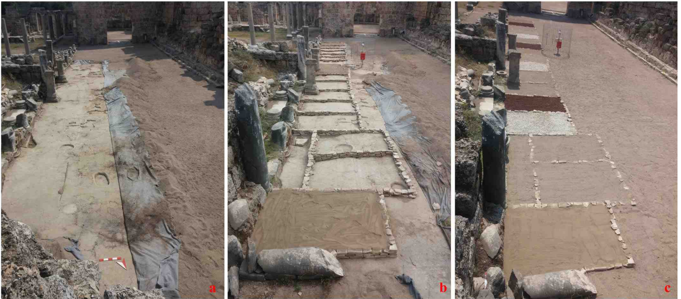
Figure 3 Installation of Monitoring Station, Test Areas and Measuring Devices.
