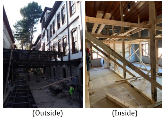
Figure 16. Scaffolding (Ankara Directorate for Surveying and Monuments, 2021).
