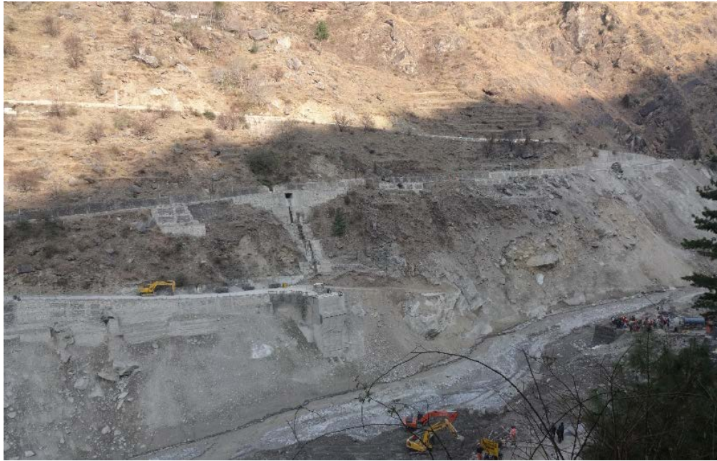
Figure 3. Washed off motorable RCC bridge over Rishiganga on Joshimath – Malari State Highway at Rini
