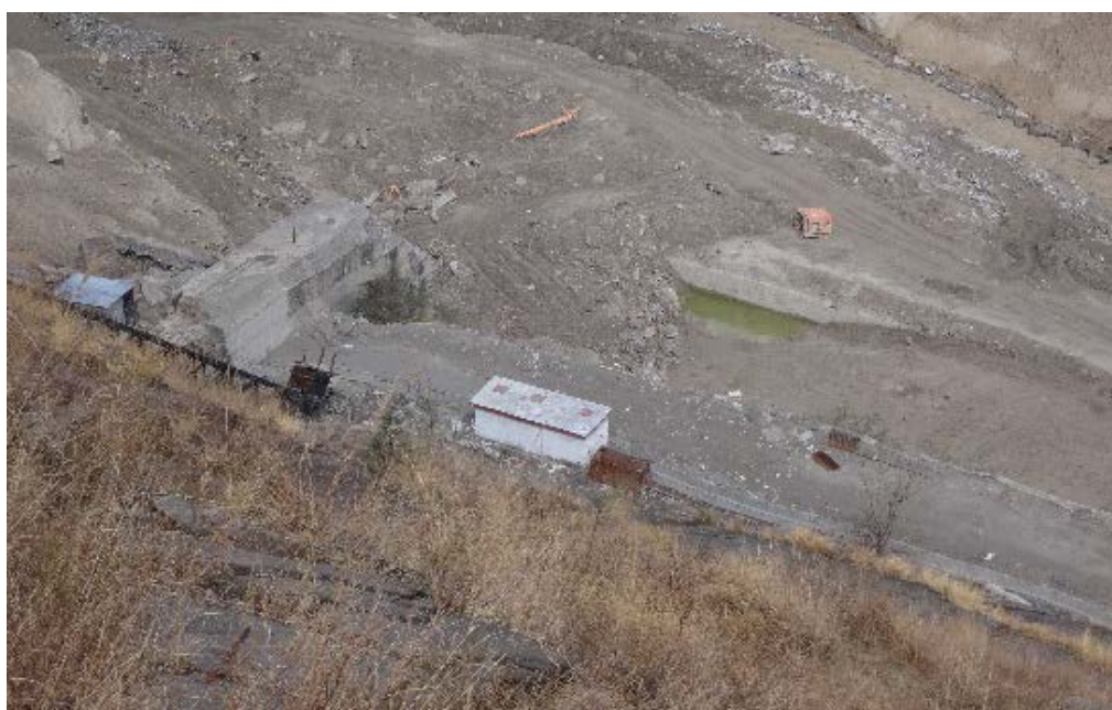
Figure 2. Washing away power house of Rishiganga hydropower project of 13.2 MW capacity upstream of Rini
