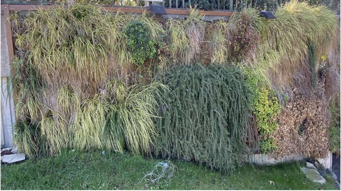
Figure 3. The vertical garden application in IDO Vehicle Exit Underpass
