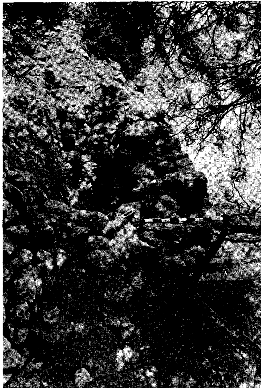
Fig. 25 — Pre-Hellenistic Defense Wall on the Acropolis. Section through core and east face. Looking north.
