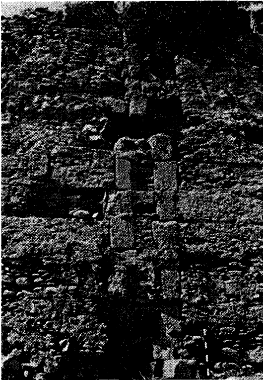
Fig. 33 — Detail of Mixed Masonry and Cemented Rubble Construction. Theatre, Western Parodos Wall, Pier 6.
