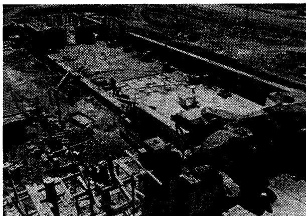
Fig. 25 — Main Hall and Forecourt of Synagogue after structural repairs, September 1970. Looking east.
