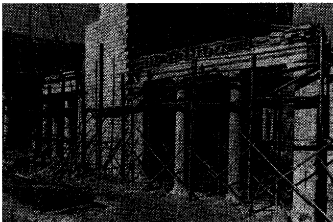
Fig. 31 — Entrance to North Hall (Hall 'BEN') in Process of Reconstruction.
