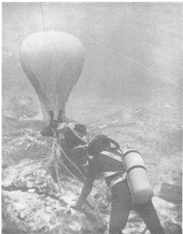
Fig. 11 — Frederic Dumas and Duthuit filling balloon with air to raise a lump of cargo.
