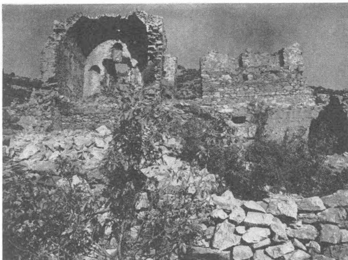
Fig. 5 — Anemurium, Tomb A II 14, East Side before Restoration.
