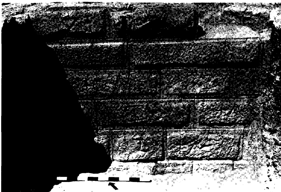
Fig. 28. Sector MMS-N, Lydian East Wall, sandstone masonry, looking northeast.
