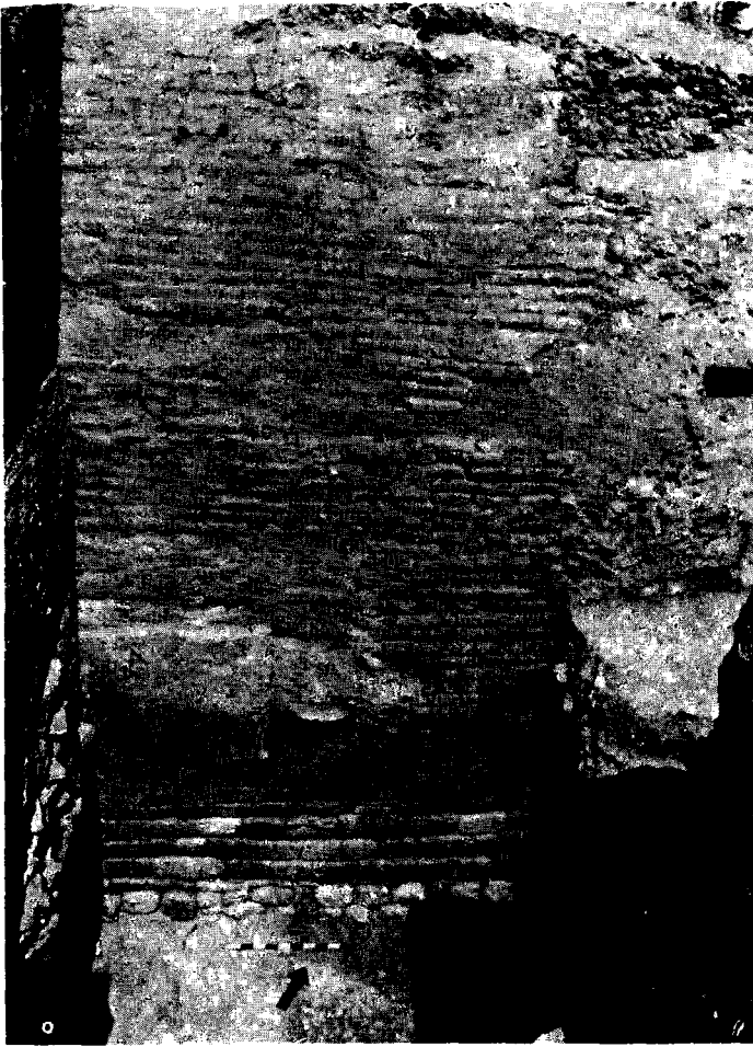
Fig.: 4 — «Colossal Lydian Structure,» sloped (east) face of coursed mudbrick with stone socle
