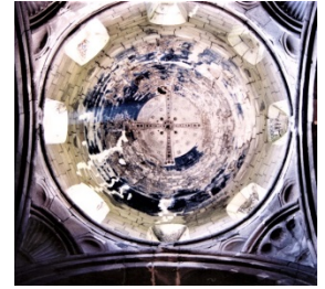
Fig. 72. Hahuli Kilisesi, kubbe
