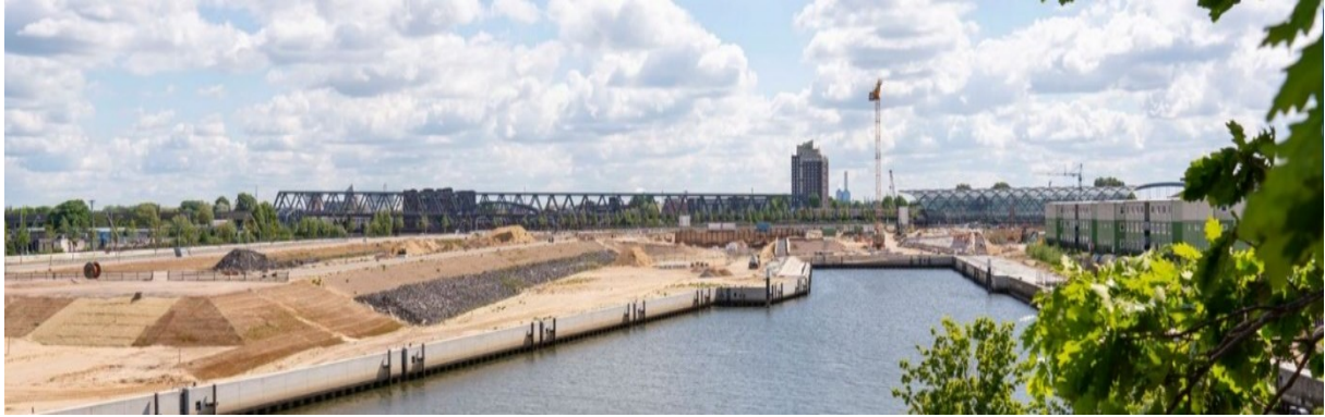
Resim 8: İnşaat alanı ( https://www.hafencity.com/en/urban-development/infrastructure )
