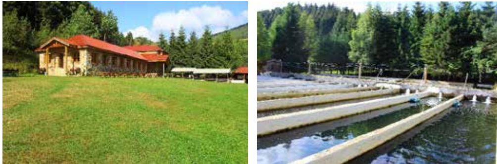
Figure 12. An Aquaculture Facility in Mountainous Areas of Giresun.
