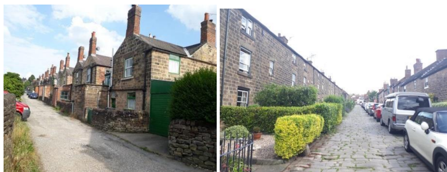
Figure 9.a-b. The 18th and 19th-century millworkers' houses, the Long Row, Belper
