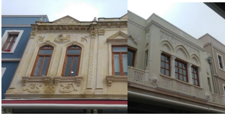
Figure 13. Facades of some of the Uzunçarşı shops-2 April 2, 2018.
