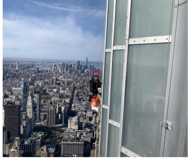
Figure 2. Maintenance work on the facade of the building (Mattani,2020)
