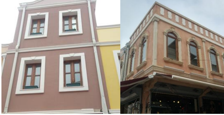
Figure 12. Facades of some of the Uzunçarşı shops-1 April 2, 2018.
