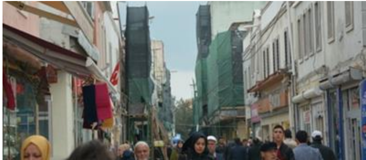
Figure 16. 1st Stage of the restoration in 2017 (Balci, 2017, May 5).
