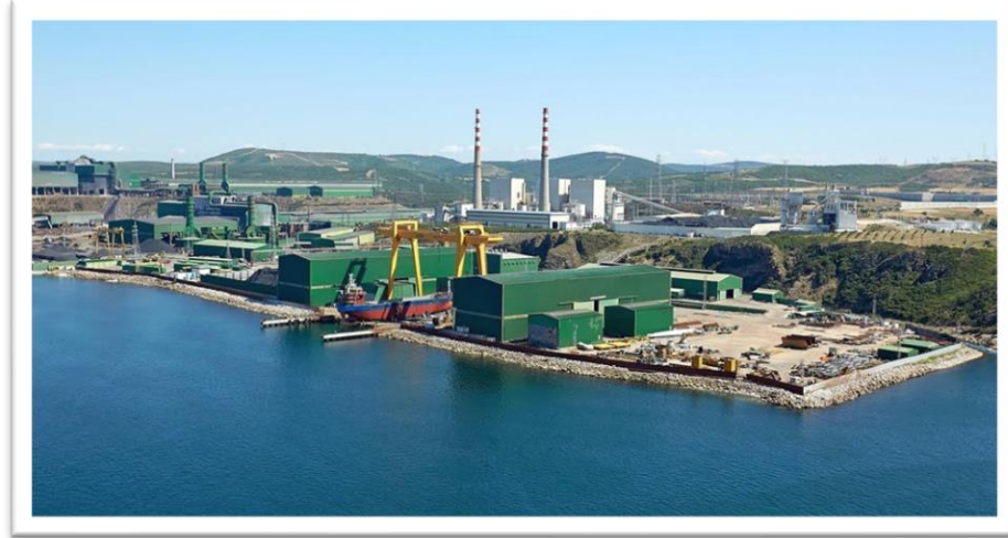
Photo 6: Biga İÇDAŞ Steel Energy and Shipyard Factory ( https://www.youtube.com/watch?v=F4KAtbB1YgE )
