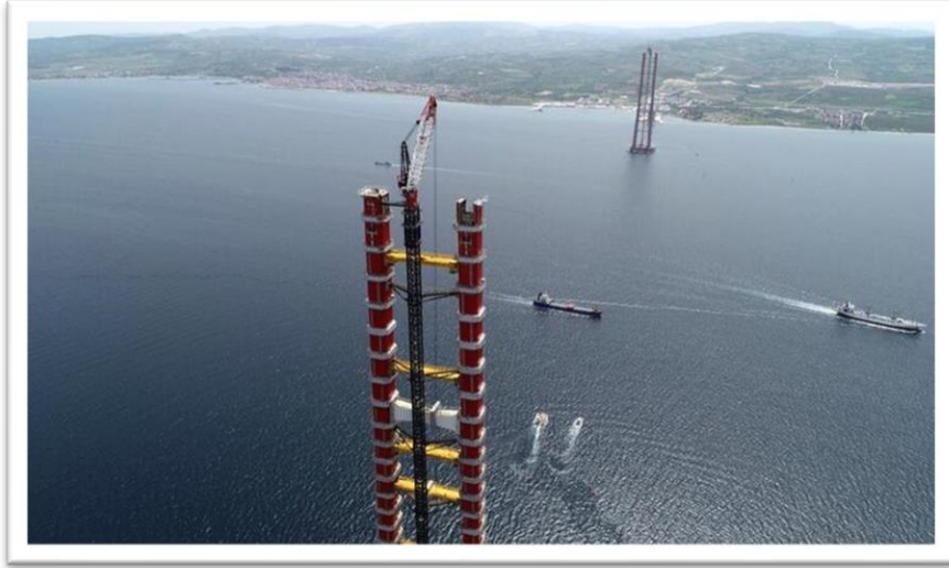
Photograph 1: Feet of 1915 Çanakkale Bridge ( https://www.canakkalehaber.com/1915-canakkale-koprusu-nde-kedi-yolu-yapimi-eylul-de-basliyor/5518/ )
