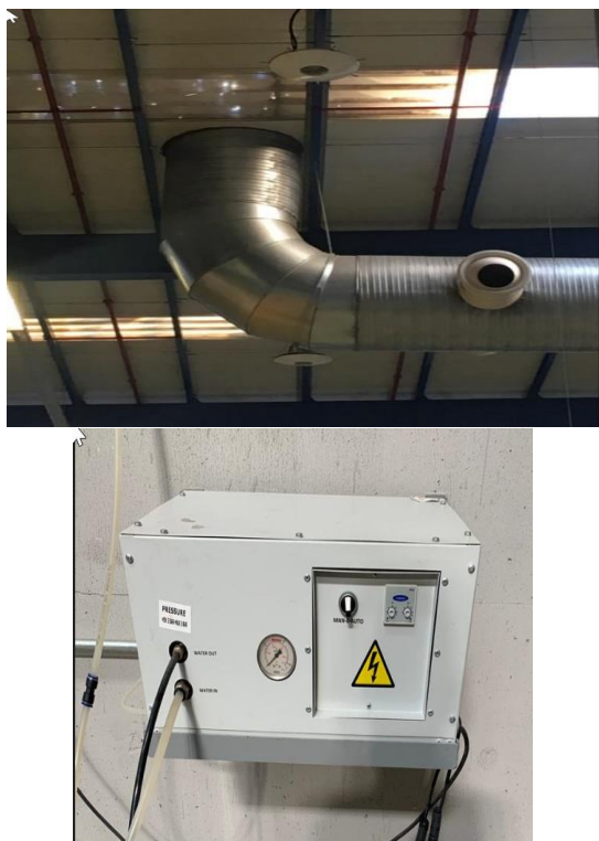
Figure 6. (7x0.17mm ) Pulverized spraying equipment and pump assembly
