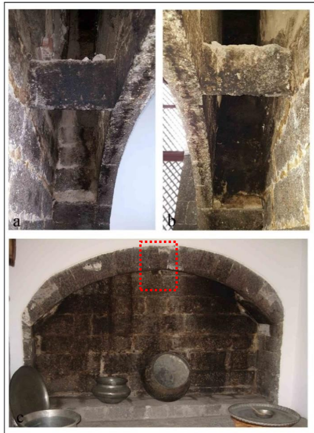
Figure 15. Binding support stone
