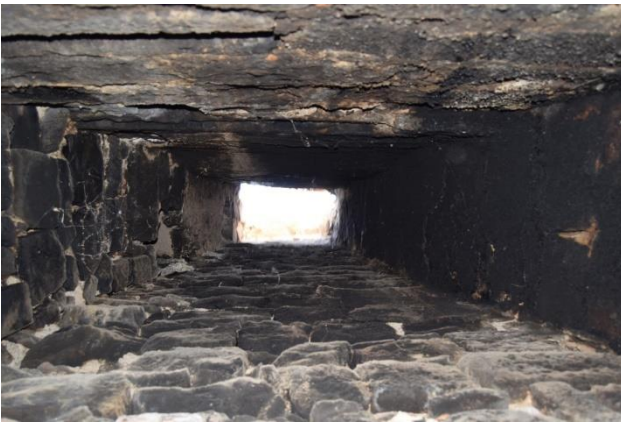
Figure 13. A view from inside the chimney
