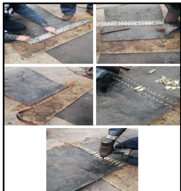
Figure 8. Images of the mechanical splicing application
