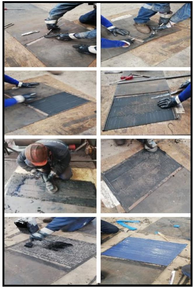
Figure 4. Images of belt splice preparation stages
