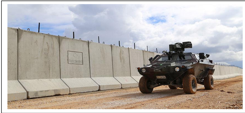
Figure 1. The Construction of a Concrete Barrier on Turkey's border with Syria. 8
