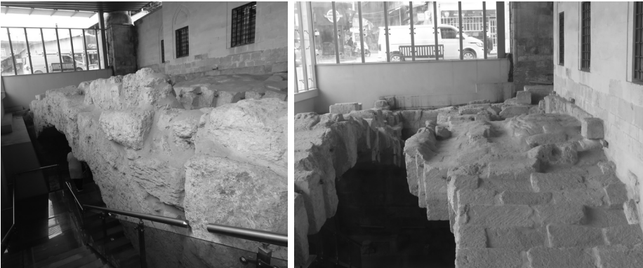
Fig. 2-3 General View of the Downstream Façade of the Bridge and the Top View of the Vault (Photo: İlkey Göçmen).
