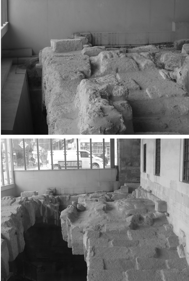
Fig. 10-11 Detail of the Cart Ruts in the Deck of the Bridge (Photo: İlkay Göçmen).
