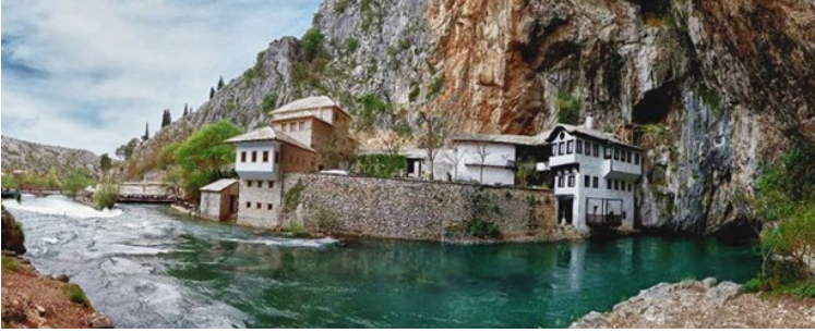
Figure 4: Panoramic view of Blagaj tekke
