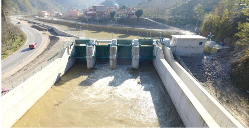
Figure 1. Yumrutepe HPP Regulator Area
