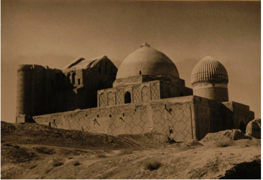
Figure 12: East facade. Photo of 1951 Mankovskaya L. Photo album to the report on the architectural and archaeological study of the mausoleum of Khoja Ahmed Yasawi during the restoration of 1951-1959. Code number 16,1971.
