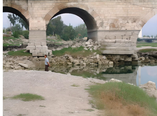
Fig. 7. Cutwater in the West from the Downstream Façade
