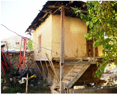
Fig. 2. An Example of a Granary with a Residential Function Above it in the Village of Elmalı Gölova
