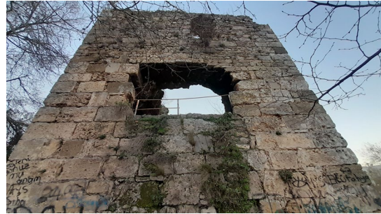
Fig. 4. Bastion Structure East Facade
