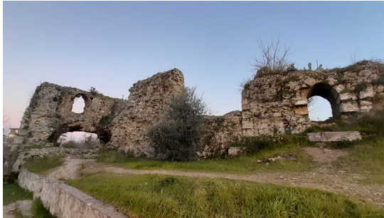
Fig. 3. Roman Fortress North Facade and Bastion Structure
