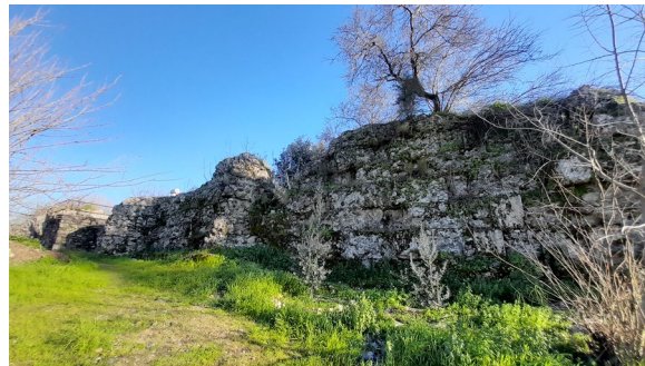
Fig. 7. Roman Fortress North Facade
