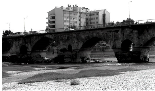
Fig. 6. Arches to the East from the Upstream Façade
