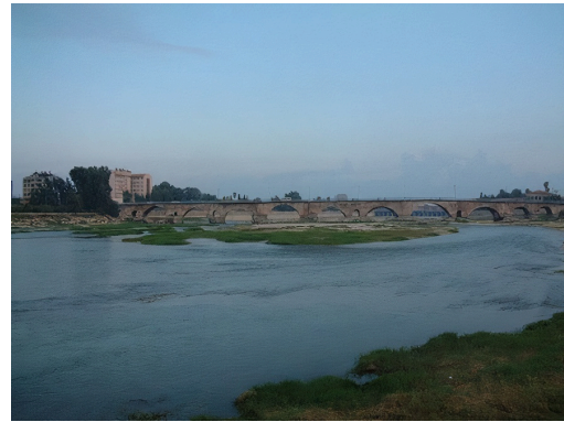
Fig. 5. General View from the Upstream Façade of Taşköprü
