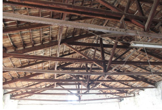
Fig. 14. Roof Construction of the Soap Factory Building (Photographed by Interior Architect Elif Türkmen)
