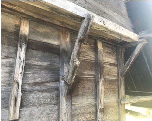
Fig. 15. Wooden Pillars and Roof Support Units
