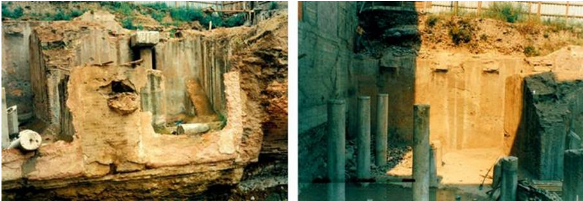
Figure 4. Antic Hotel Excavation During Construction (Antic Hotel Official Websites, 2022)
