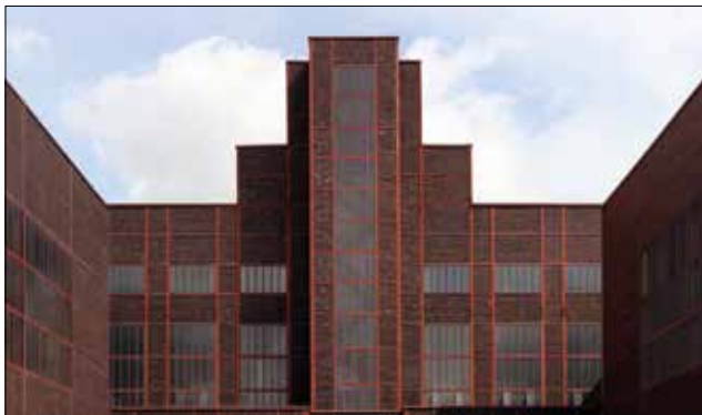
Fotoğraf 9: Zeche Zollverein Eski Kazan Dairesi ( https://thelink.berlin/wp-content/uploads/2017/11/Zeche-Zollverein-02-%C2%A9-Hendrik-Bohle.jpg ) / Zeche Zollverein Former Boiler Room
