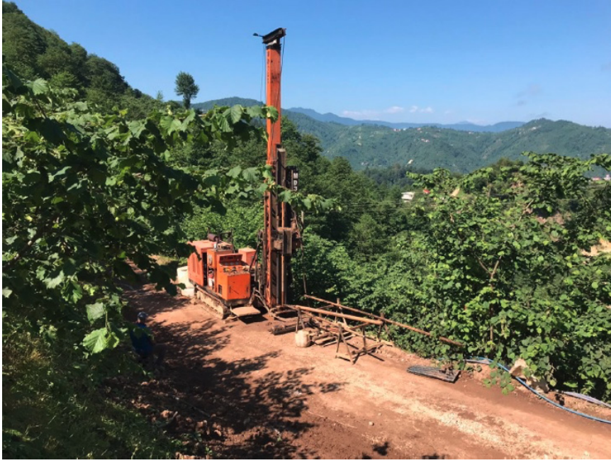
Figure 11. Core drilling at the site
