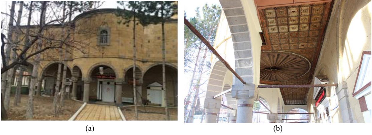
Figure 1. Ferteck Church (a) front facade (b) narthex ceiling
