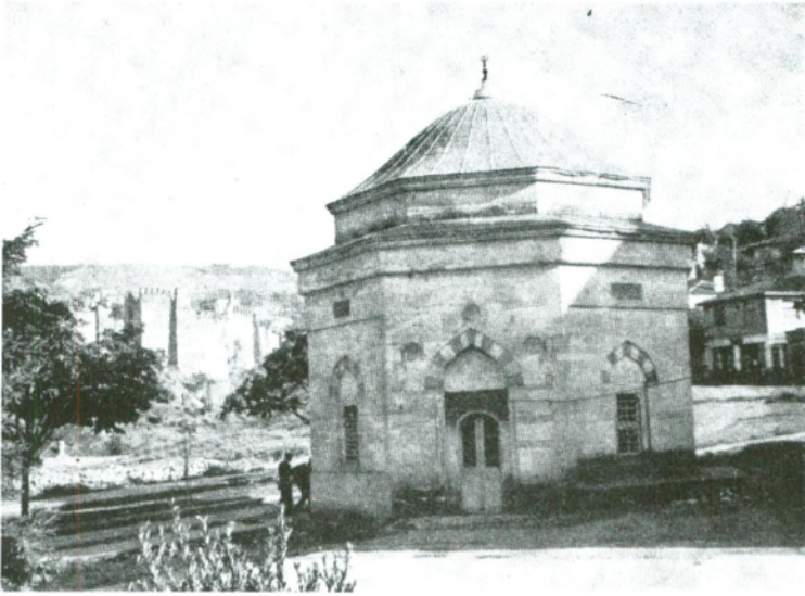
Fig. 4 — Türbe of Gülbahar Sultan, from the north.
