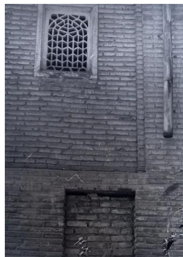
Figure 15. The entrance of the Chilakhana in an old photo. It was closed at the last restoration study (Madaniy Meros Agentligi, 2022)
