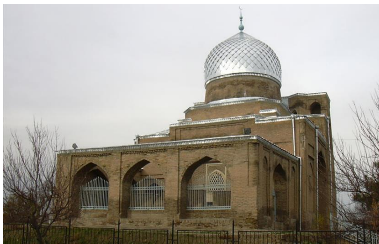
Figure 13. Facade (Backside) of Abubakr Kaffal ash-Shashi Tomb and metallic covers on the dome after an earthquake (1920-1991); It looks like a Russian style church.
