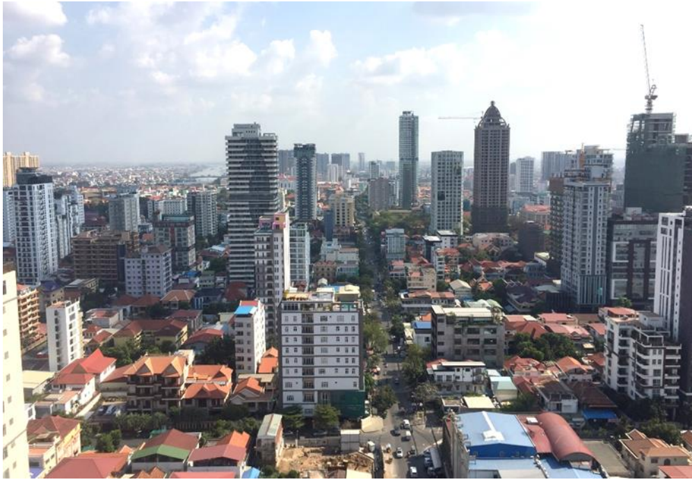
Figure 9. High-rise buildings emerging in the Central BKK1 Neighborhood, Phnom Penh.
