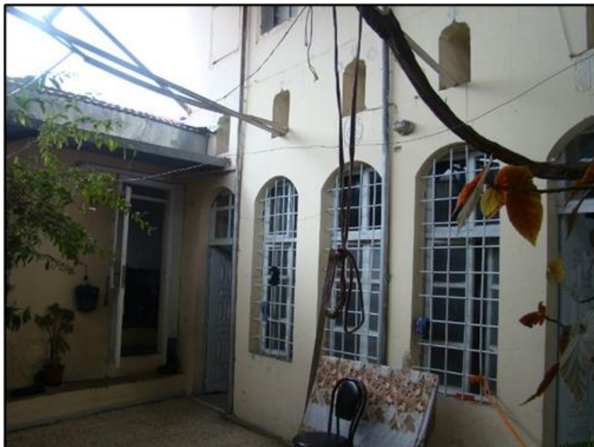
Figure 5. The courtyard-main mass-annex building relationship in the close vicinity
