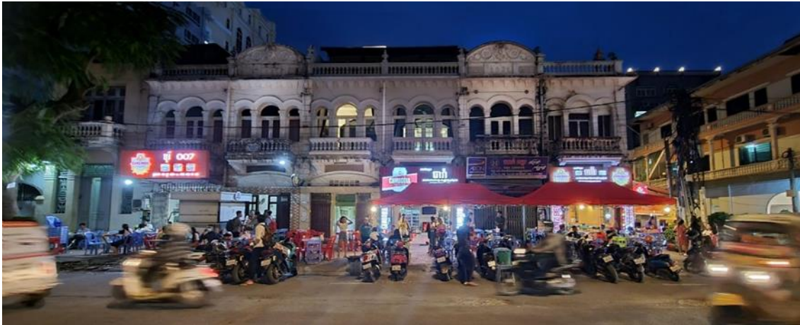
Figure 6. Old Chinese Shop Houses Front, Phnom Penh.
