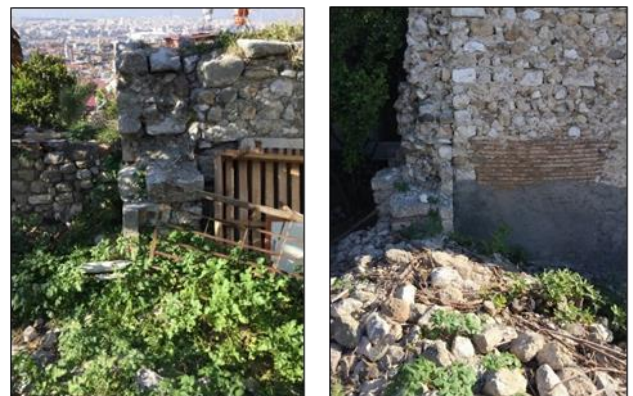
Figure 17. Traces confirming the existence of the door-window opening of the mass, which could not reach the present day, in the southwest of the building lot.
