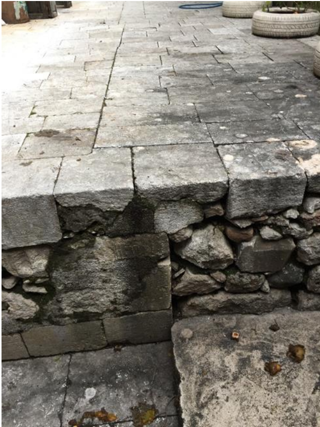
Figure 10. The photo shows that the ground level of the First Period was lower and there was an access to the stone floor of the courtyard by steps after the cut stone finish
