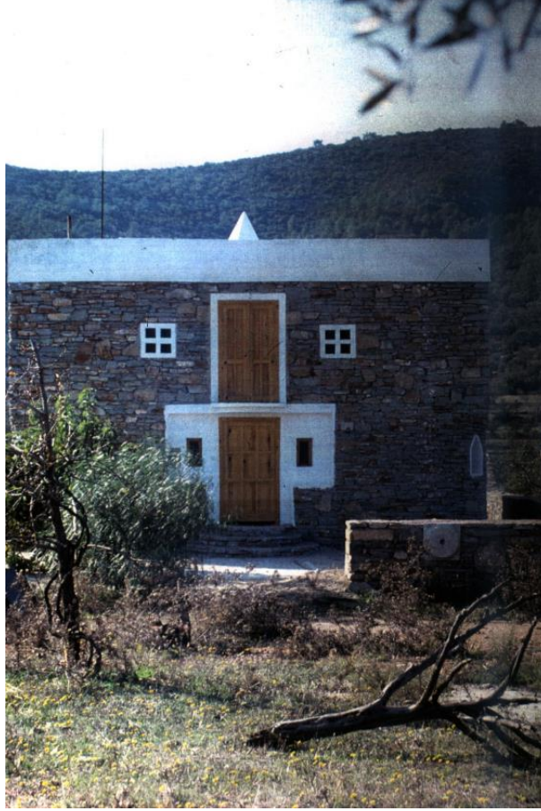
Şekil 2. Yula Evi Cephesi ( Arkiv, 2022a ) Figure 2. Facade of Yula House ( Arkiv, 2022a )
