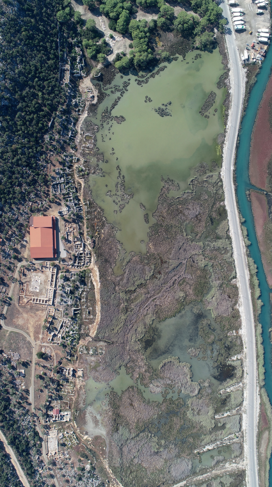
Fig. 7. Andriake. Southern Sector. Air photo. 2020.
