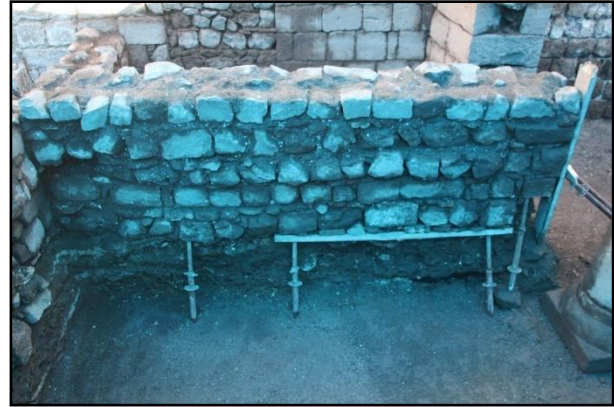
Figure 7. Basalt stone walls between 150 and 200 cm
