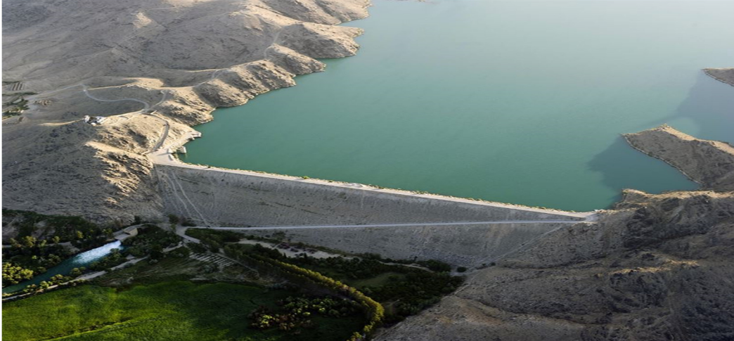
Figure 2: Arghandab Dam, Helmand, Afghanistan
