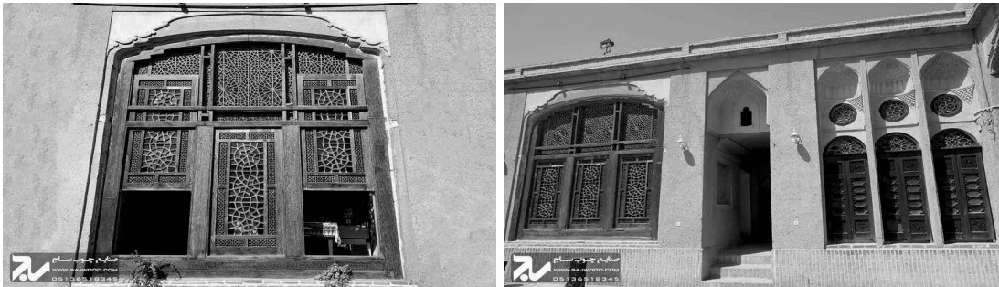
Figure 9. Traditional wooden window facing the courtyard (Orsi)
