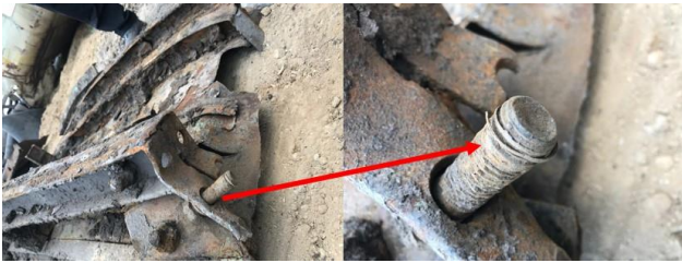
Figure 11. Nut stripped of its threads in damaged gallery lower segment.
