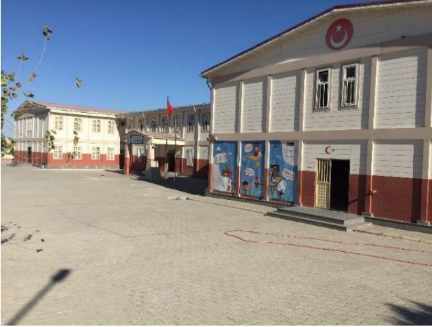
Figure 1. General view of the school building considered in the study
