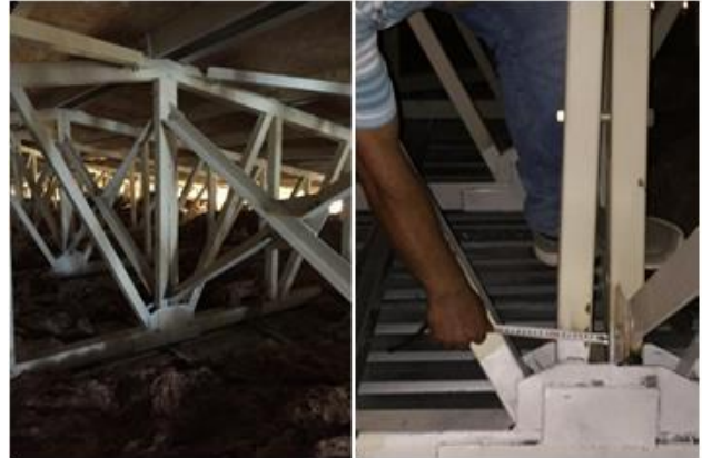
Figure 2. Roof trusses manufactured in two parts
