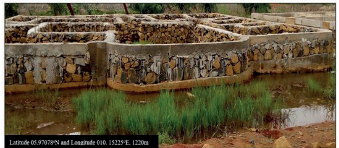
Photo 3: Rocks used for a foundation in the Mulang wetland (Field Survey, 2020).
