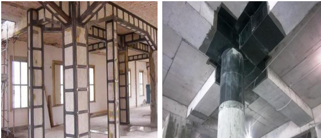
Figure 3. Reinforcement of beams
