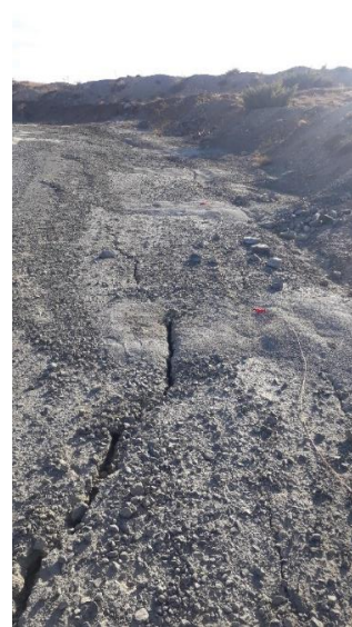
After Blasting (Second Blasting)
