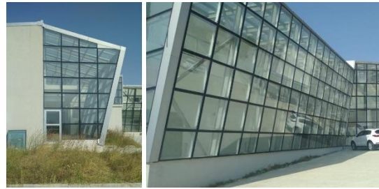
Figure 4-5. Building Exterior View
